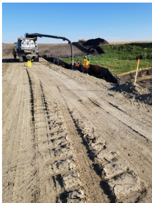
Crews working to repair and reinforce Riparian buffer at SSKP 1018 Photo taken facing East
