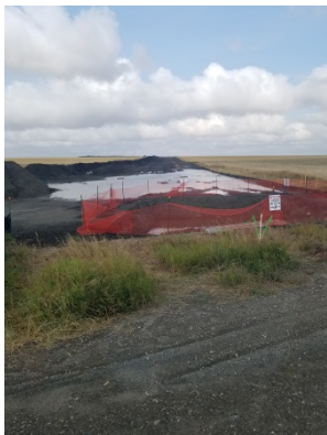
Standing water at Shoe-fly 7 Picture taken facing West
