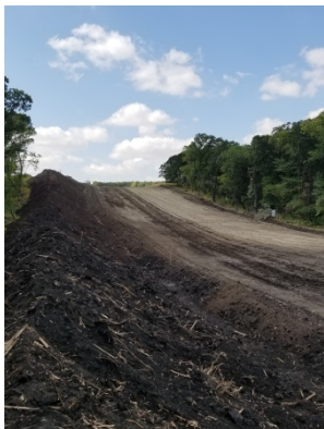
View of the escarpment facing west Location SSKP 1026
