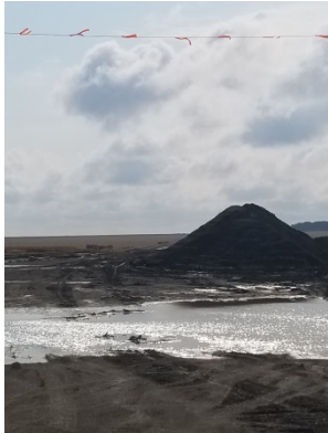
Standing water at Shoe-fly 4 Picture taken facing East
