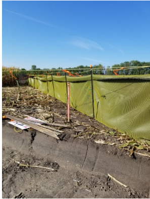
Photo of Riparian Buffer Located at SSKP 1049 Picture taken South East
